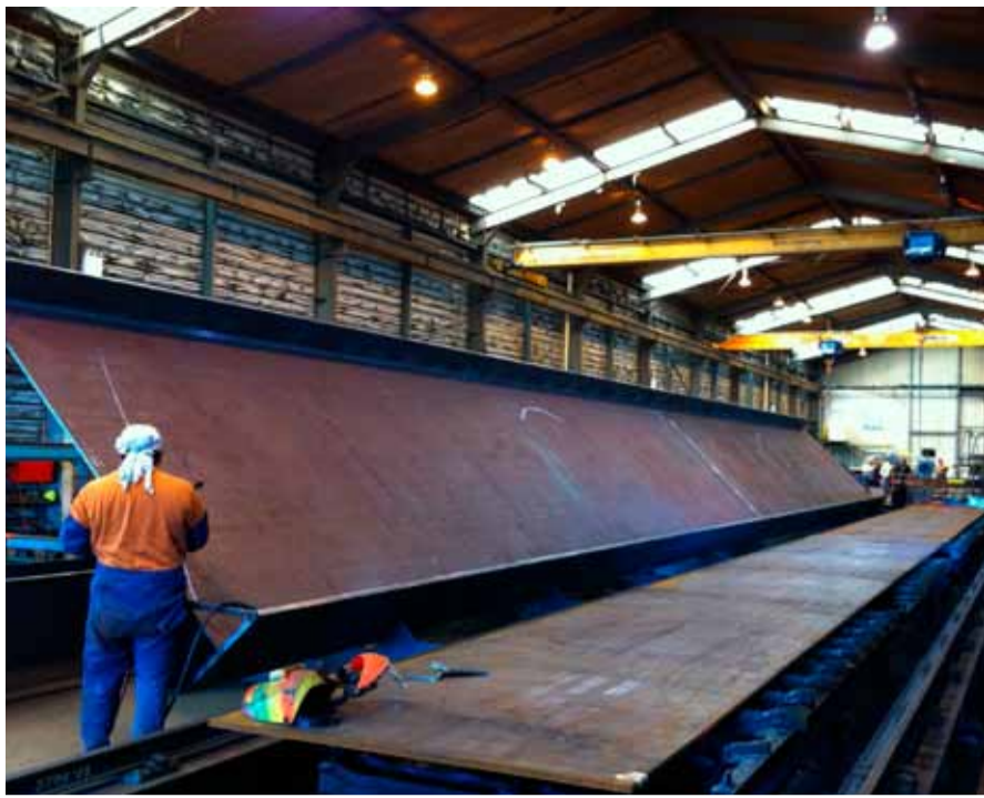
Construction of the bridge beams at Steltech workshop.
