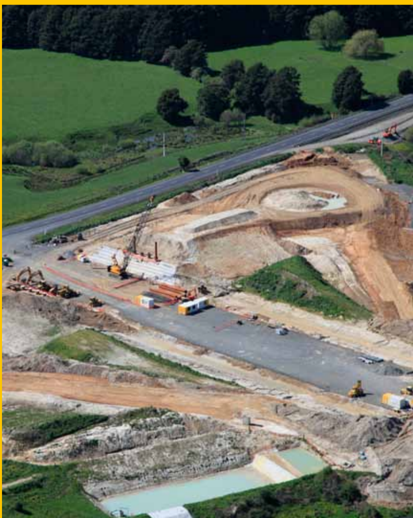
Ngaruawahia alignment looking south towards Taupiri. Image supplied courtesy of NZTA.
